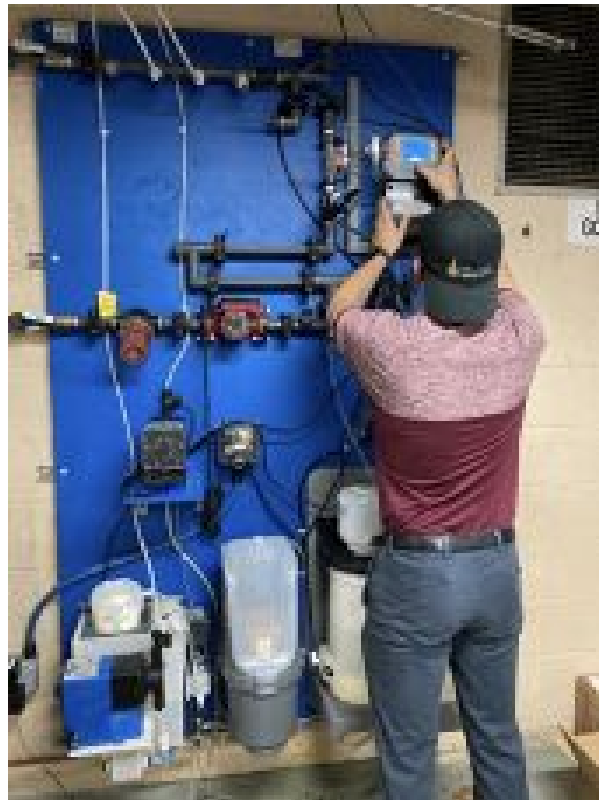
Figure 1 – Starting up a solid feed system on a tower
