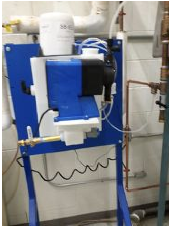
Figure 3 – Oxygen Scavenger Feed Station
