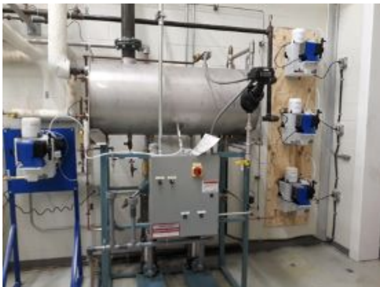
Figure 2 – Multi-product Boiler Solid Feed System
