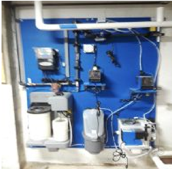
Figure 2 – Dual Biocide with Disk Feeder
