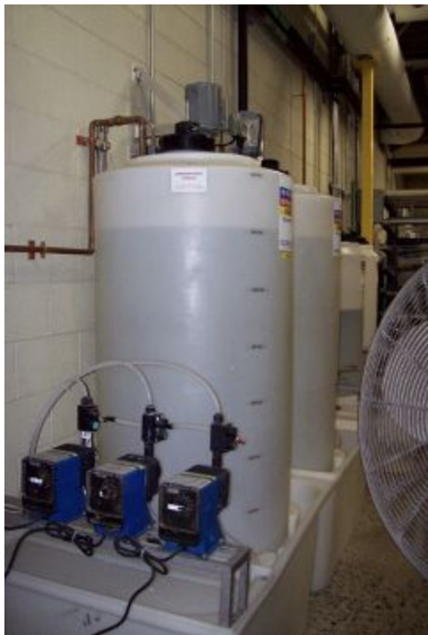
Figure 4 – Fully Automated Mix Tank Liquid Feed System
