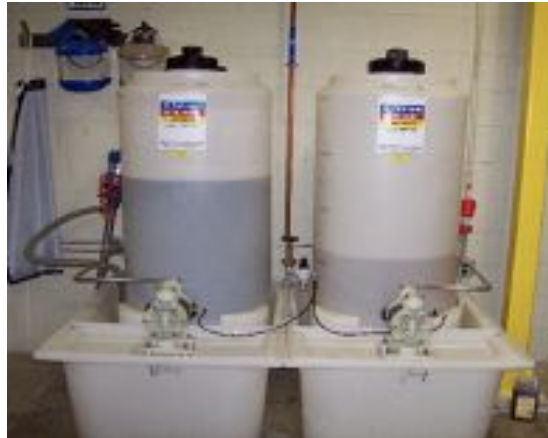
Figure 4 – Neat product tanks with containment & transfer pumps
