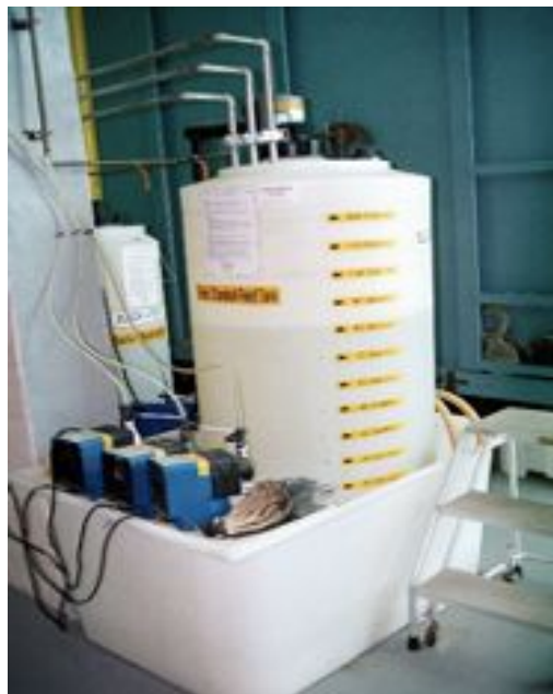
Figure 3 – Mix Tank for Automated Mix Tank System (note three (3) lines injecting neat chemical into larger mix which in turn treats three (3) boilers via the metering pumps
