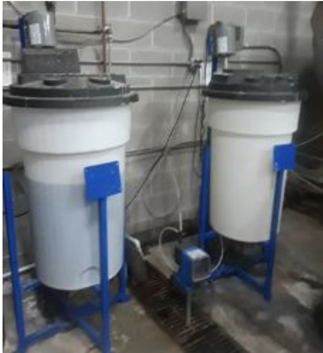
Figure 1 – Dual Mix Tank Boiler Liquid System
