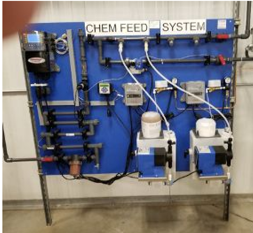
Figure 1 – Single Biocide with Inhibitor Jug Feeder
