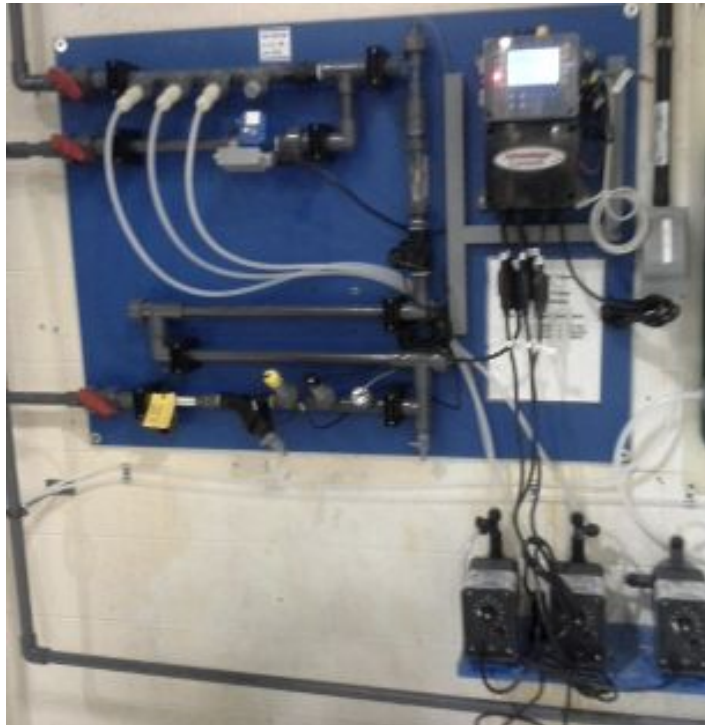
Figure 1 – Wall mount for liquid feed system
