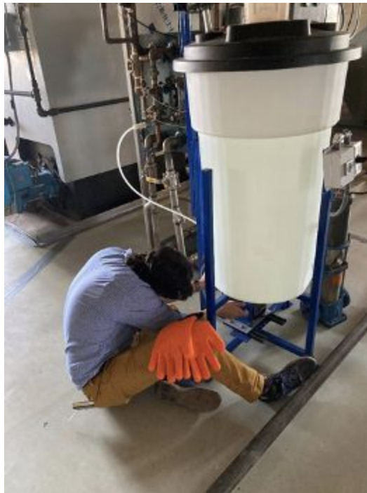
Figure 5 – Troubleshooting Mix Tank for a Liquid Feed Boiler System
