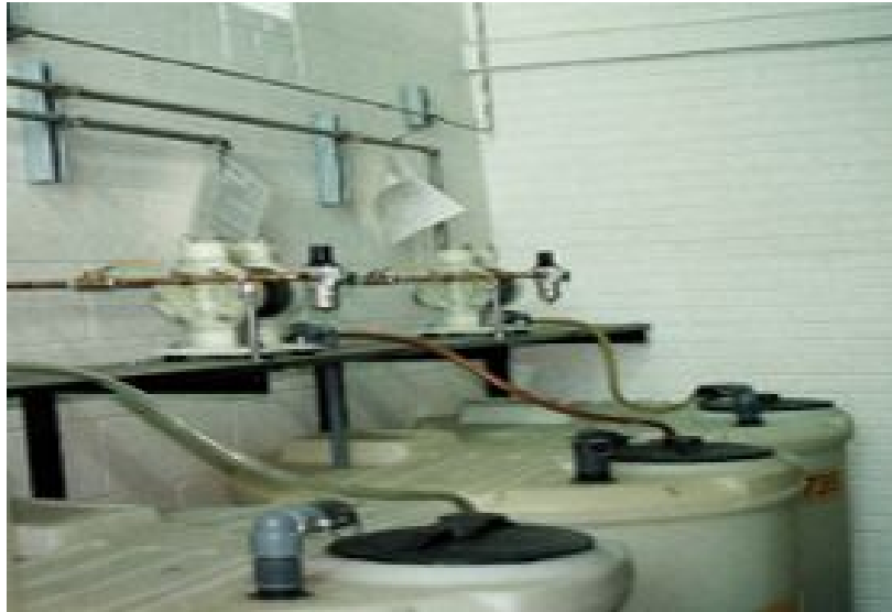
Figure 2 – Neat Tanks with Transfer Pumps for Automated Mix Tank System
