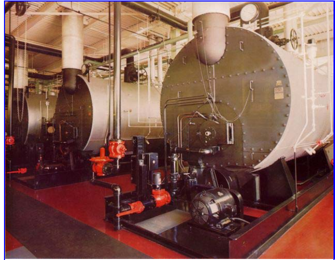
Three 1955 - 500 hp Cleaver-Brooks Boilers
